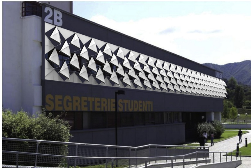
Fig. 5. Blinking sail solar façade: partially-open configuration.
