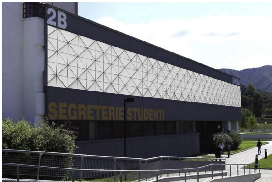
Fig. 4. Blinking sail solar façade: fully-closed configuration.
