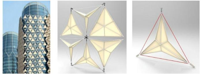
Fig. 1. Illustration of the TABS design for the origami sunscreens of the Al Bahar Towers in Abu Dhabi [14].
